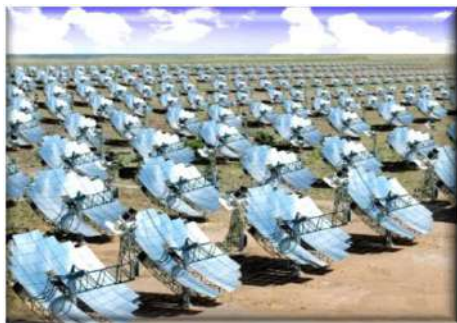
Solar Thermal Farm
